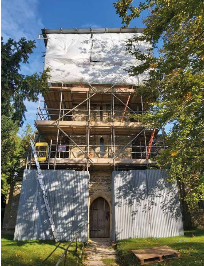
Fifehead Magdalen – tower repairs
